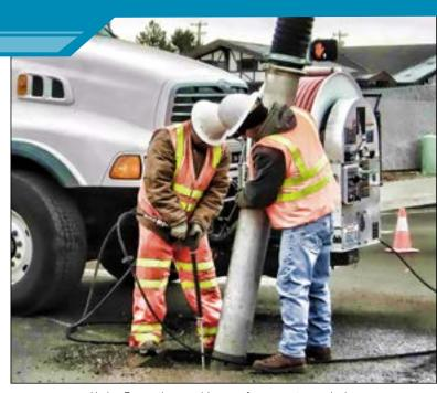
Hydro-Excavation provides a safe means to precisely excavate an area with high pressure water.
